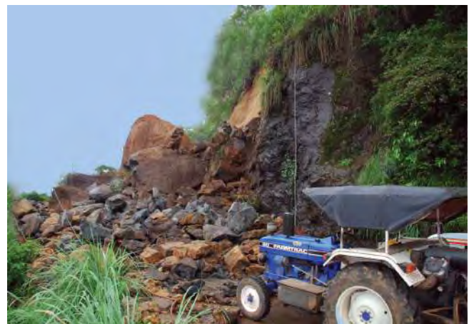
Fig. 2.1.1.3 Rock fall at Double cutting locality in the Idukki-Kattapana Road
