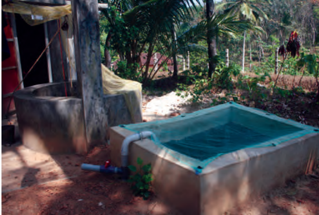
Fig.3.1.1.1 Rainwater from the roof is led into a collection tank for filtration. For this purpose, it is provided with a bed of gravel, charcoal and sand
