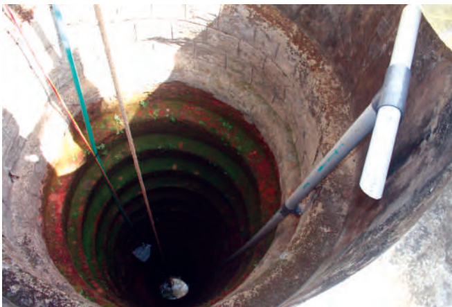
Fig.3.1.2 From the collection tank, the filtered water is led into the well. The summer rainfall of about 30 cm has enhanced the water availability in the well.
